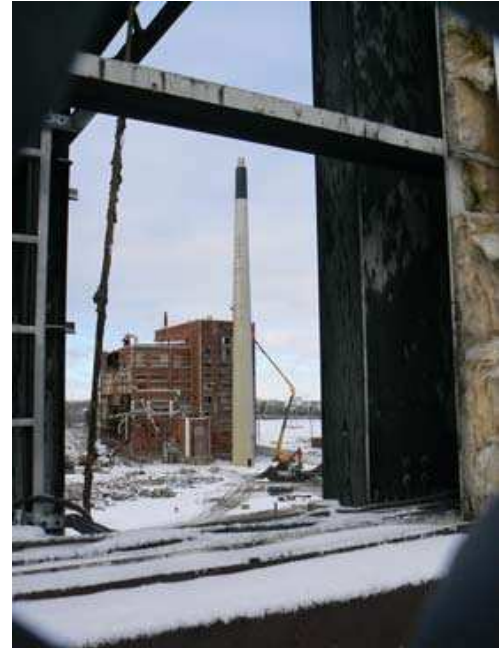
The former Domtar paper mill site offers interesting possibilities for housing and recreational lands.
